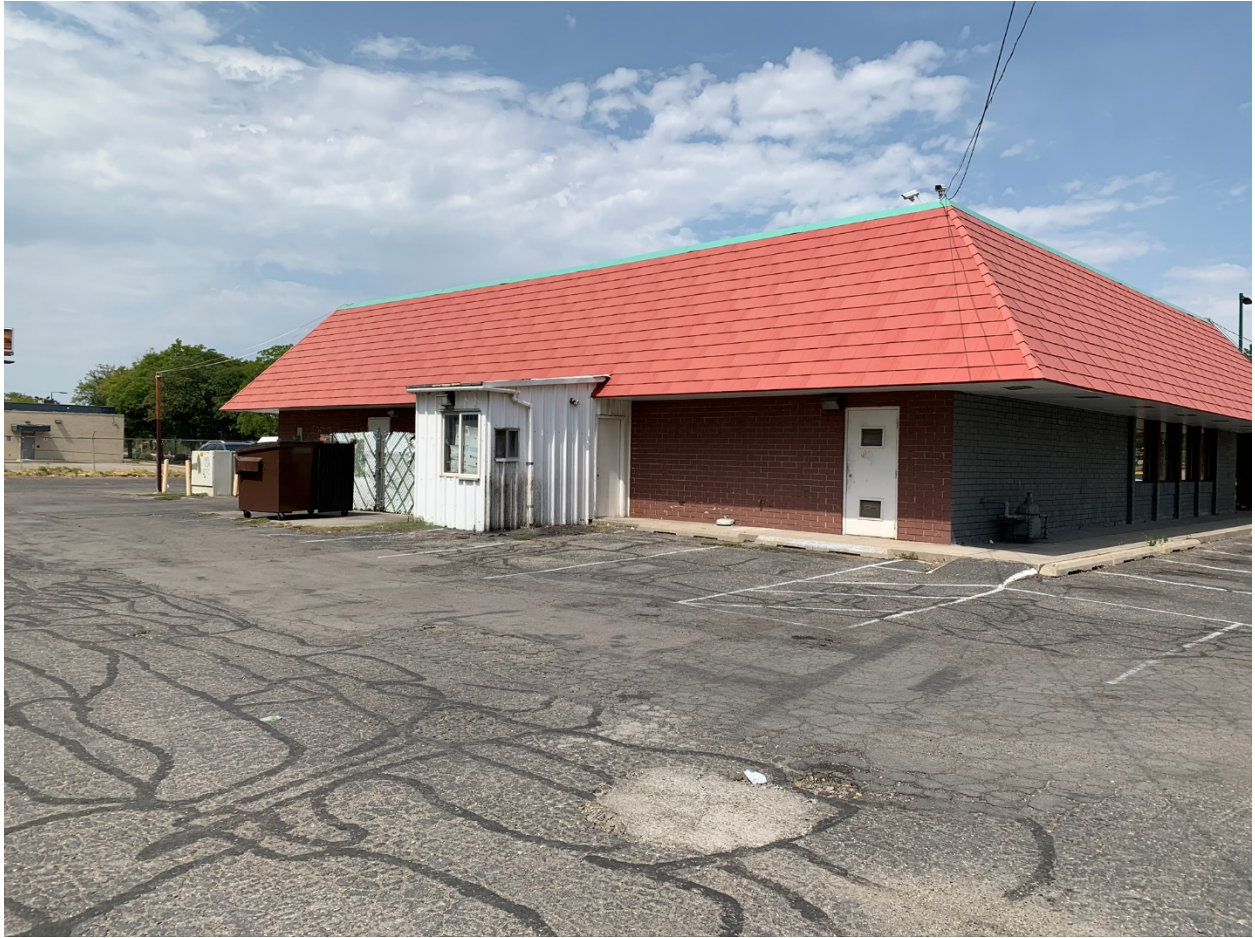
Rear view of the restaurant at 1025 W North Temple
